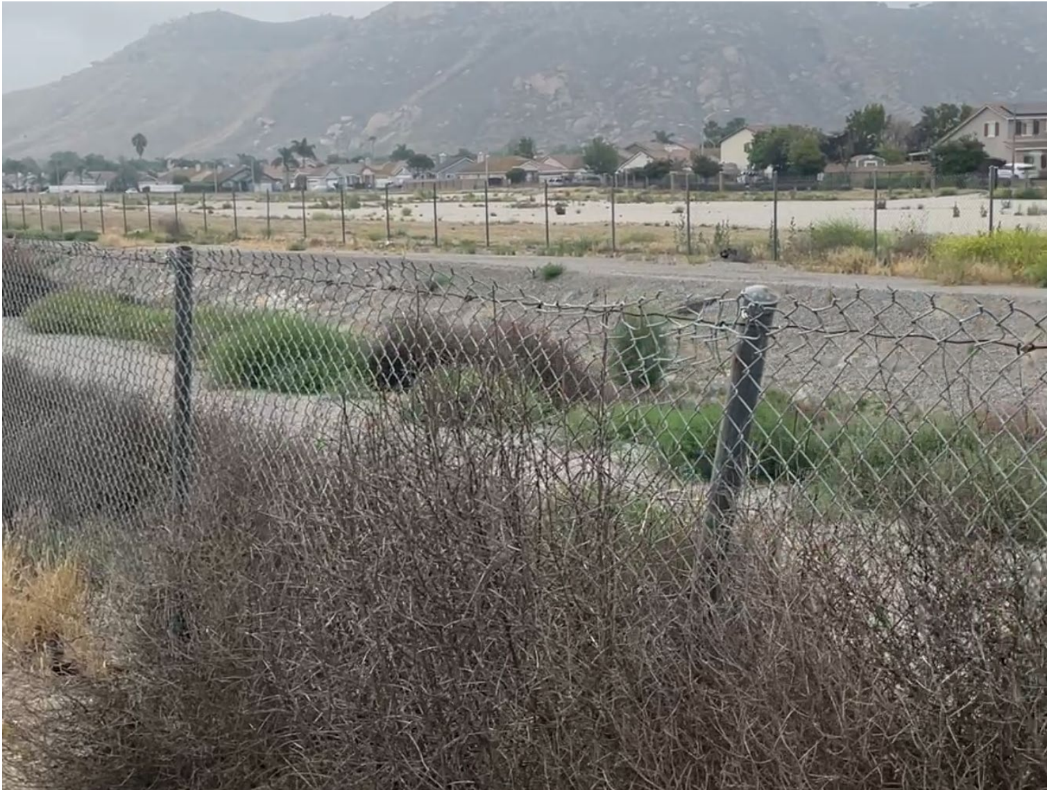
Photograph 4 - Bent fence/post at point of impact (Courtesy of FAA)
