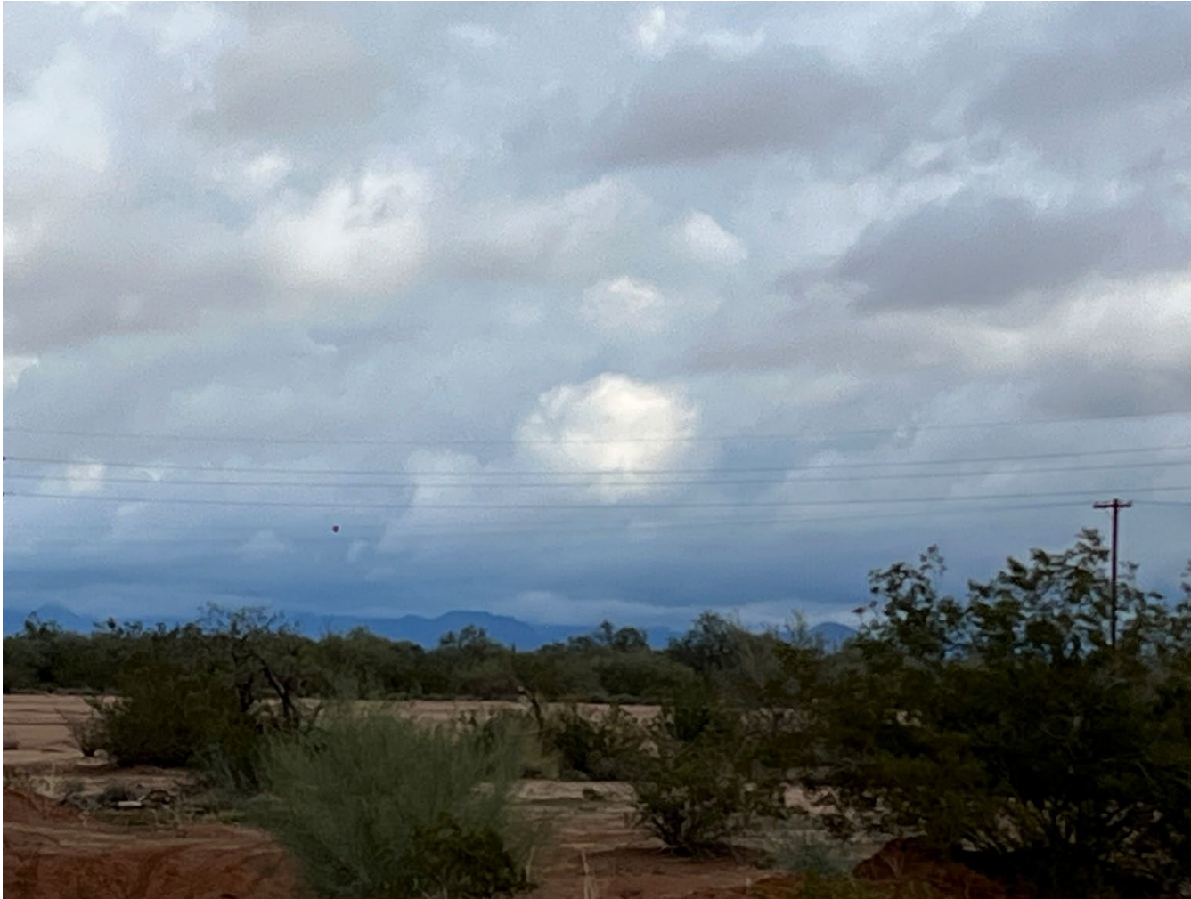
Photograph 3 - Wires struck by Airplane (Courtesy of Pilot)
