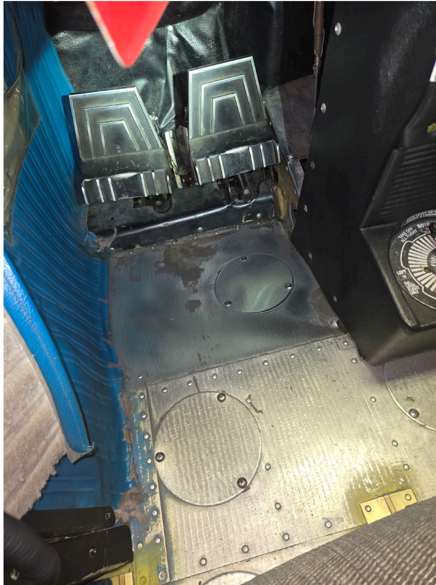
Photograph 1 - View of left side seat position fuselage damage (Courtesy of FAA)
