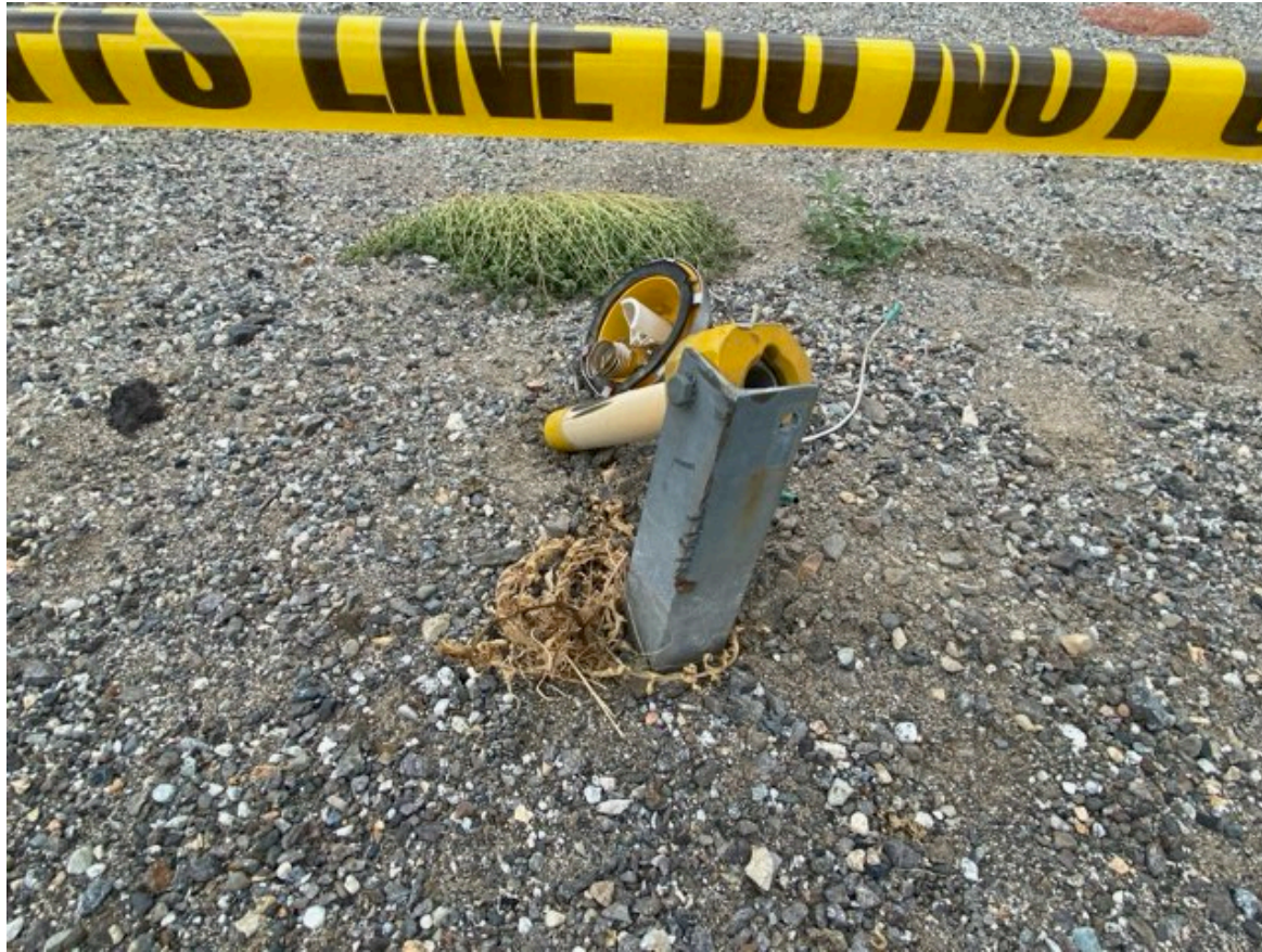
Photograph 4 - Damaged runway end light. (Courtesy of FAA)
