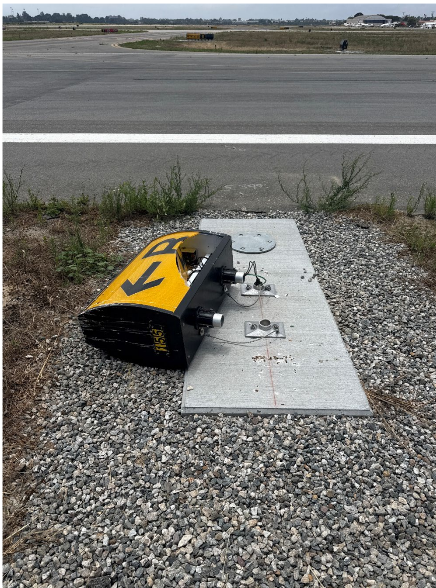
Photograph 2 - View of damaged taxiway sign (Courtesy of airport operations)
