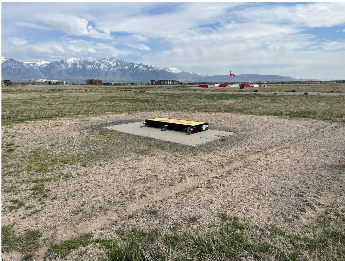
Photograph 3 - Taxiway directional sign (Courtesy of Pilot)
