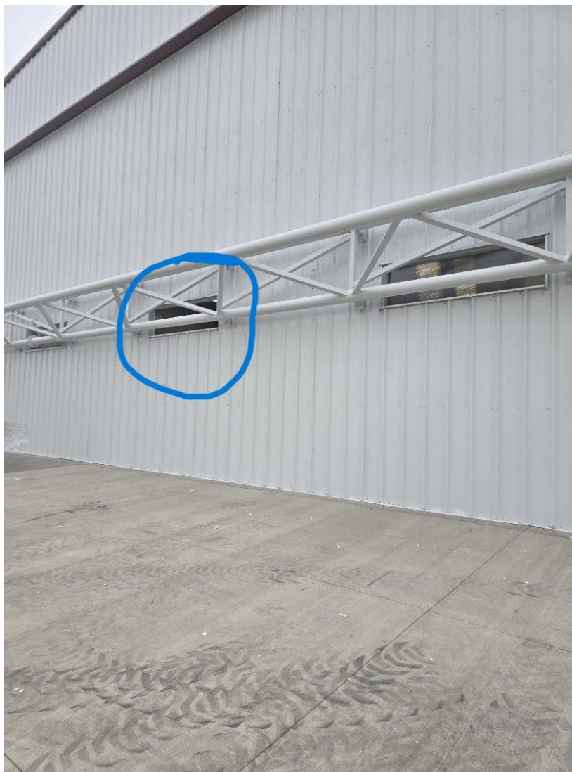
Photograph 3 - Hangar door and window. (Courtesy of the FAA)
