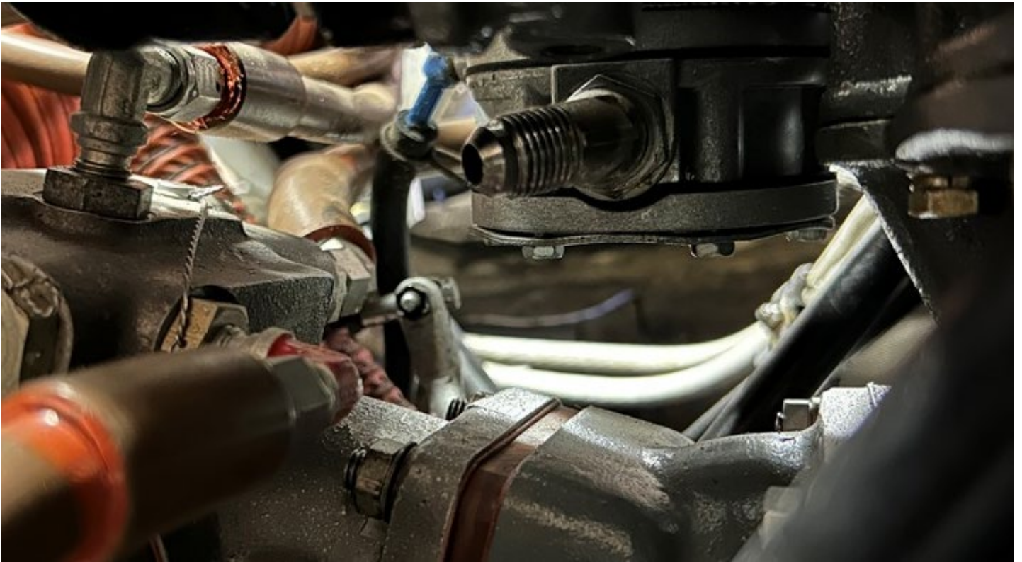
Figure 4: Inlet to pump
