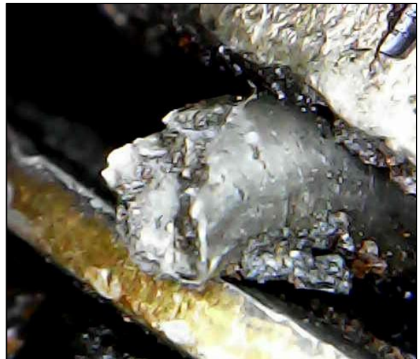
Figure 6-Mixture cable end at linkage.
