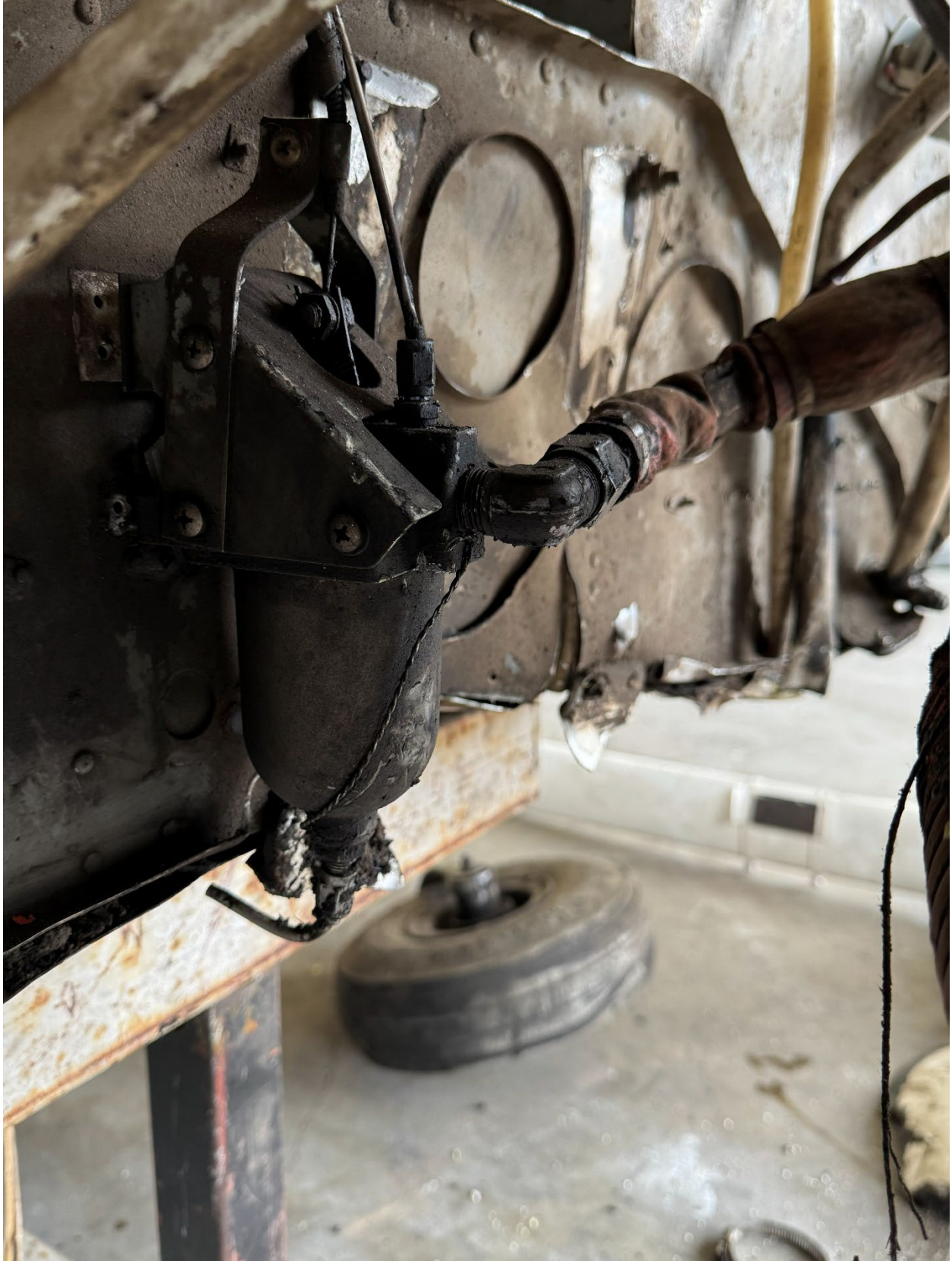
Figure 7: View of the gascolator prior to removal for examination
