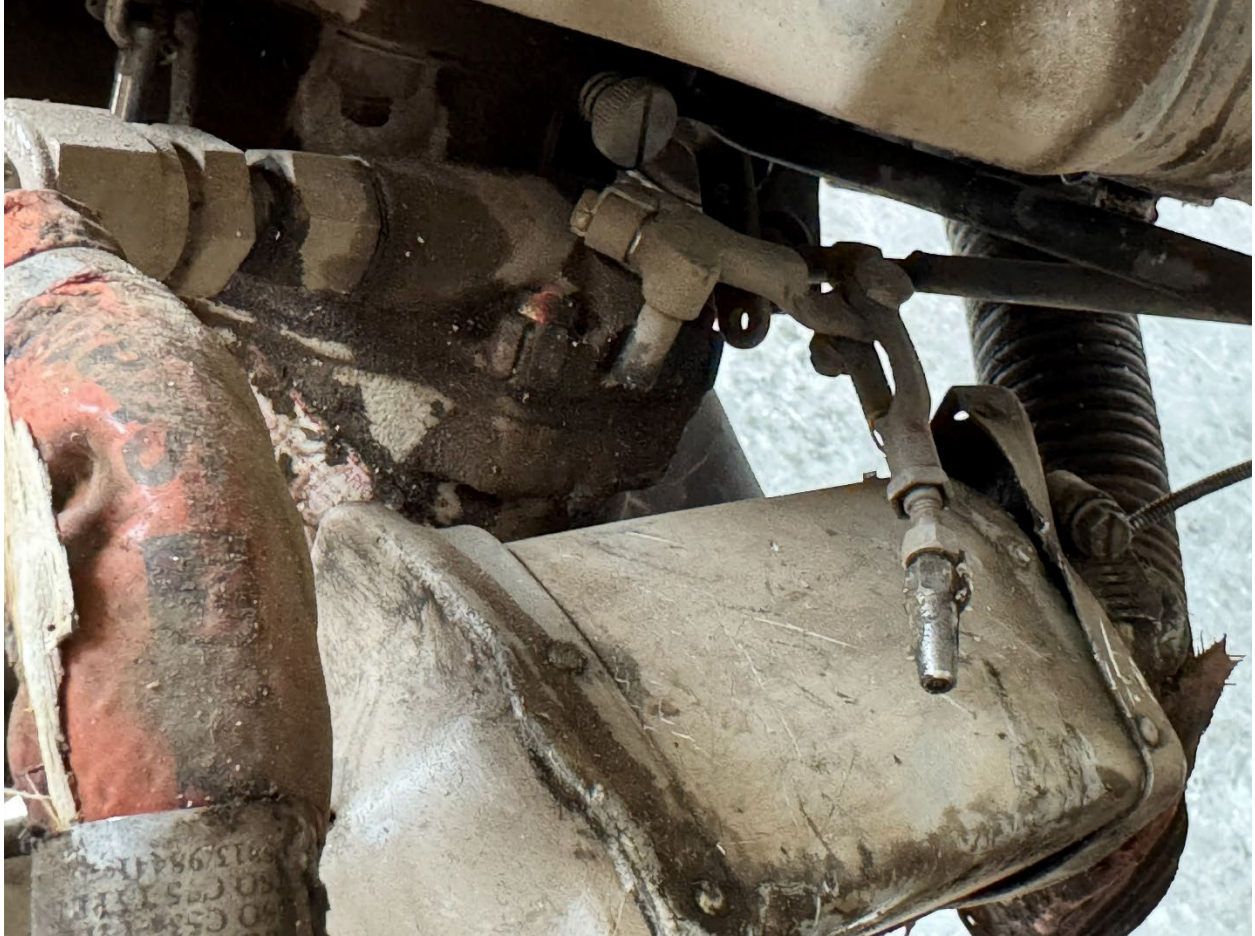
Figure 5: View of the impact damaged mixture control linkage
