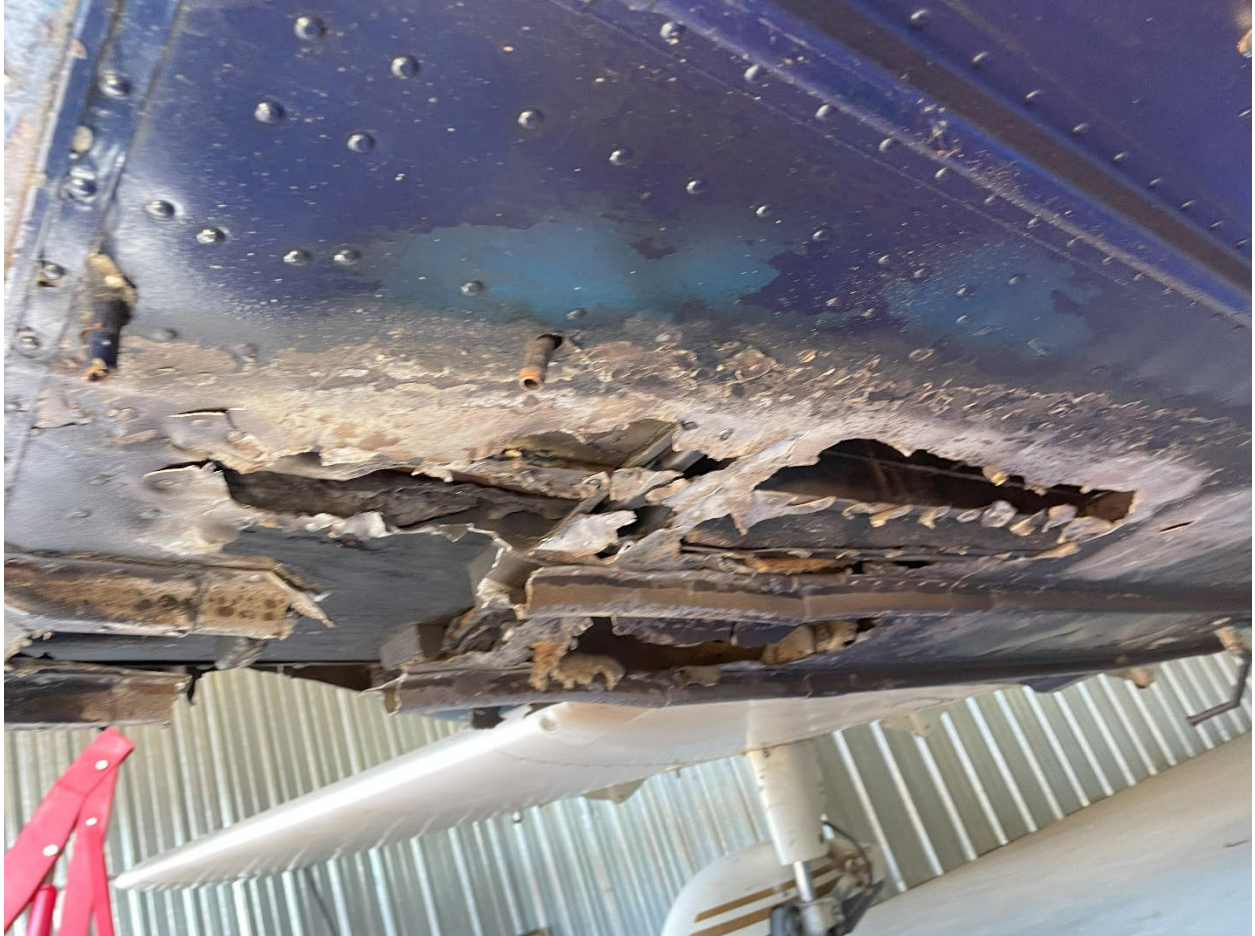
Figure 12 - View of underside fuselage fire and heat damage
