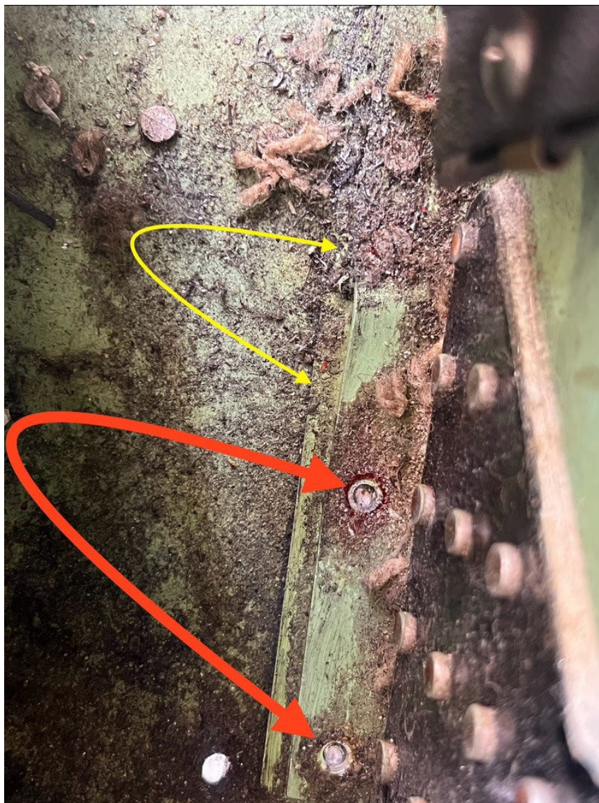
Photograph 1 - View of the damage to the left wing spar (Courtesy of operator)
