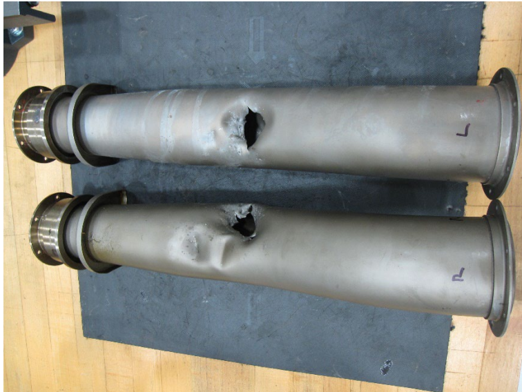
PHOTO 12: EXIT PENETRATION HOLES IN THE COMPRESSION DISCHARGE TUBES
