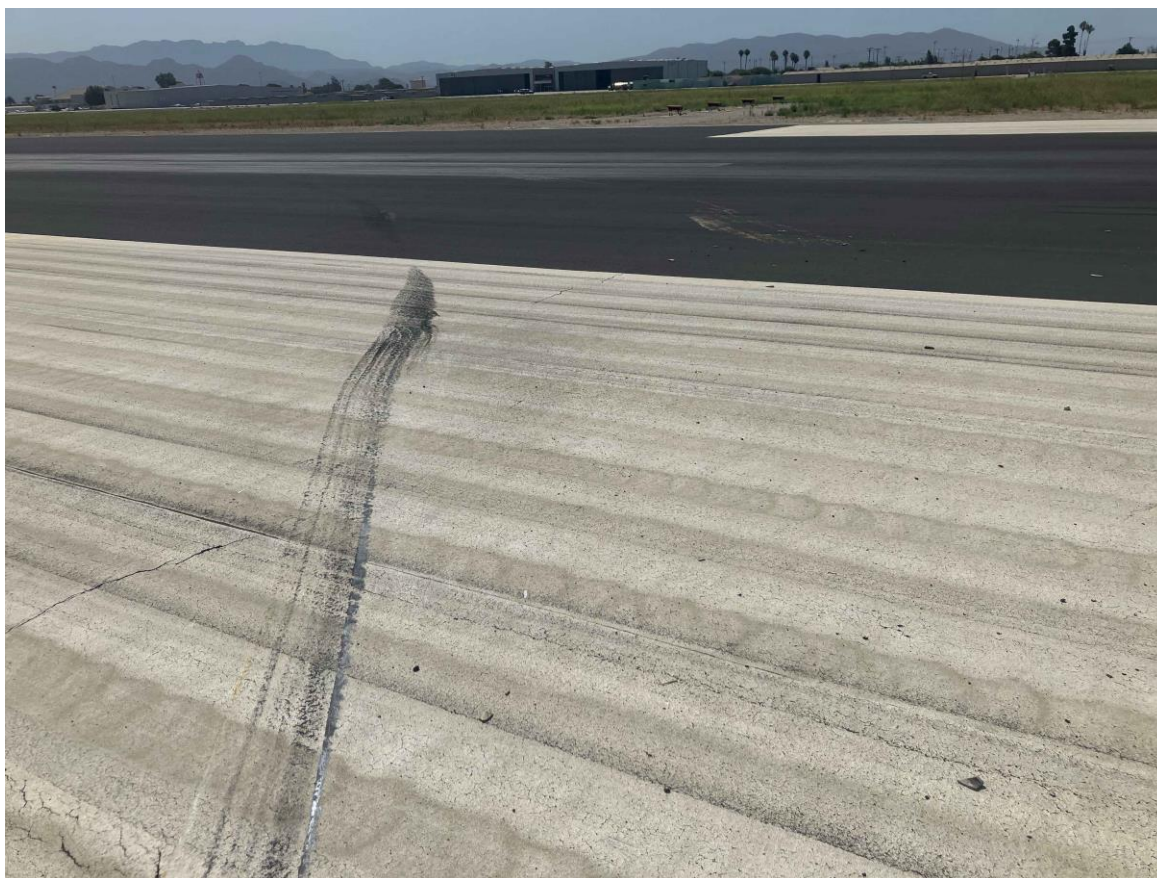
Photograph 6 - Accident site, runway impact marks. (Courtesy of CMA Airport Operations)
