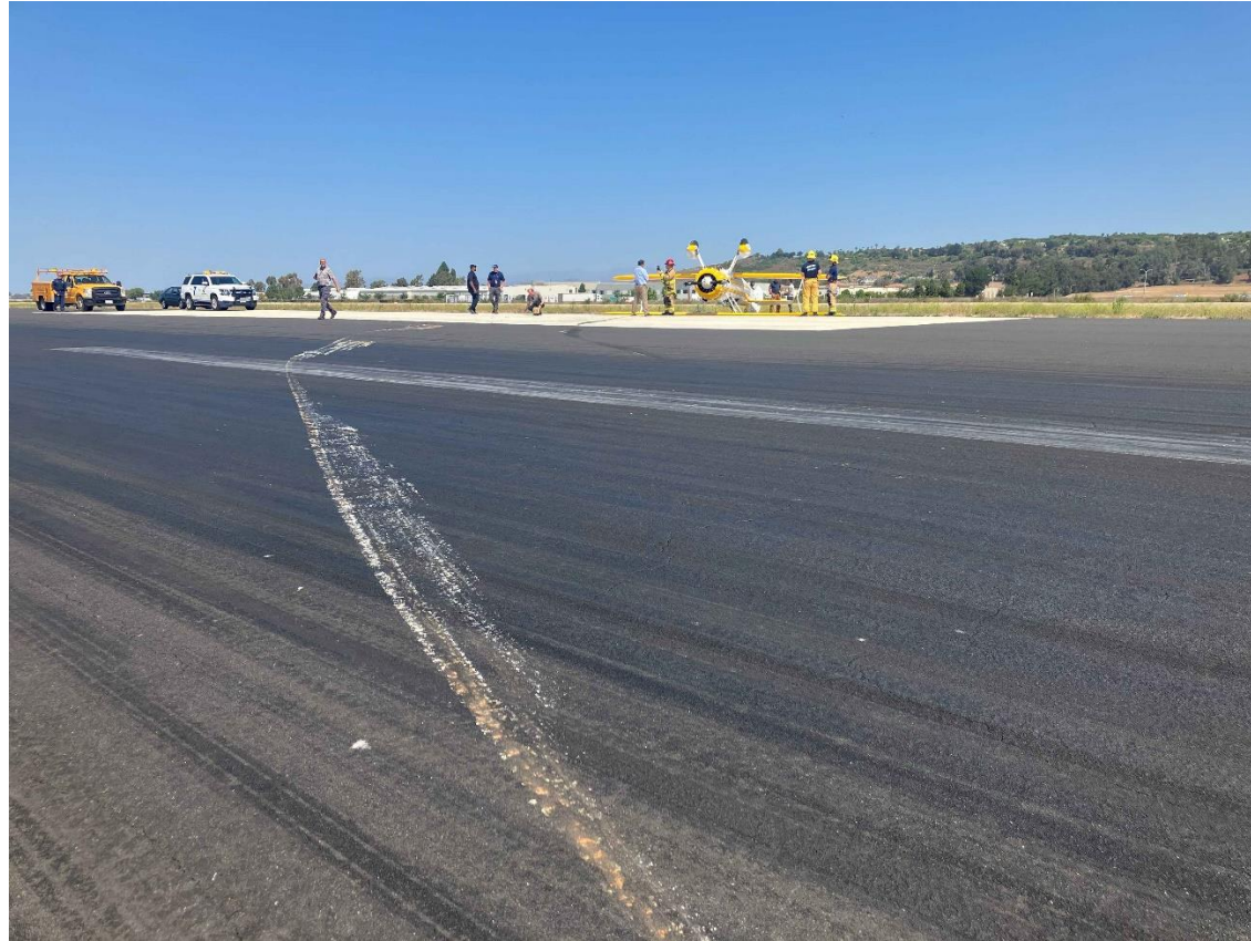
Photograph 5 - Accident site, runway impact marks. (Courtesy of CMA Airport Operations)
