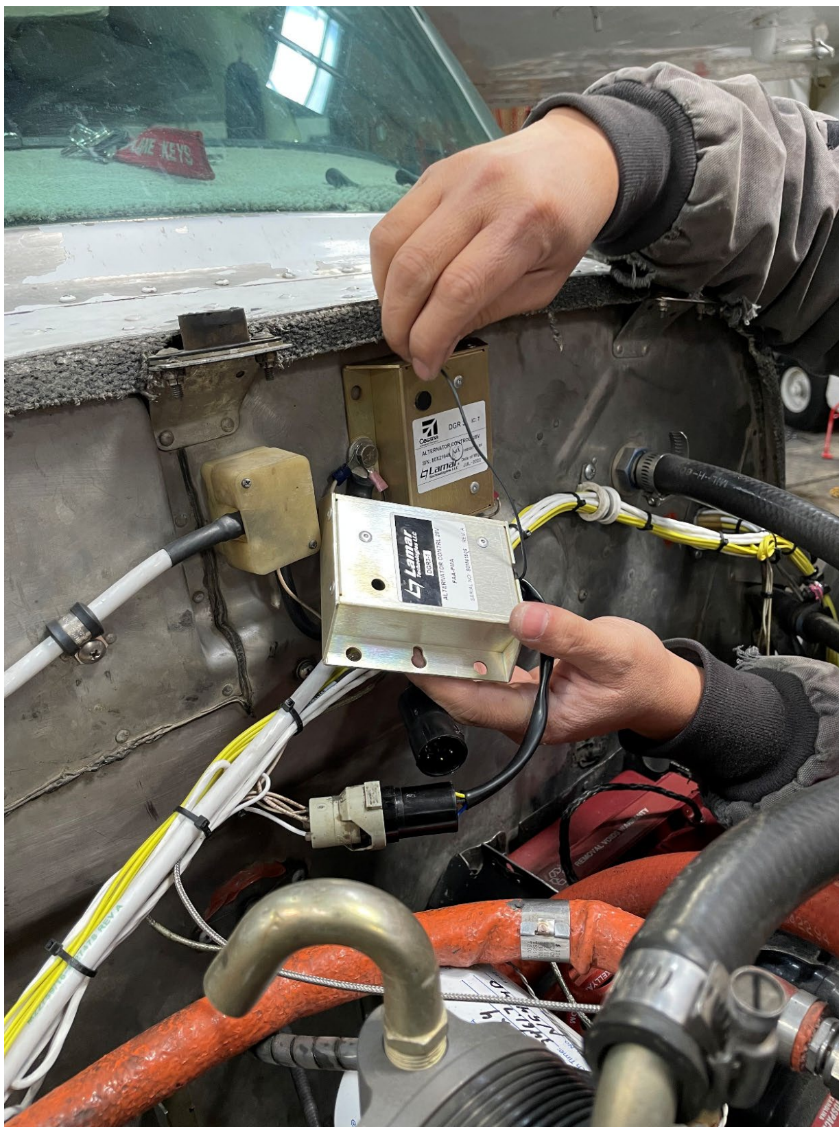
Figure 6. Accident voltage regulator alongside the exemplar voltage regulator.
