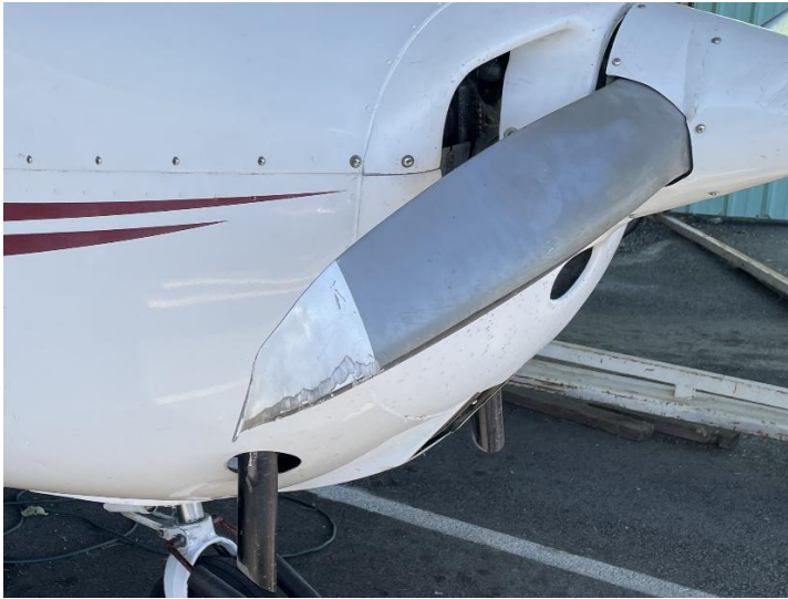
Figure 5: View of Propeller Blade Note Tip Damage
