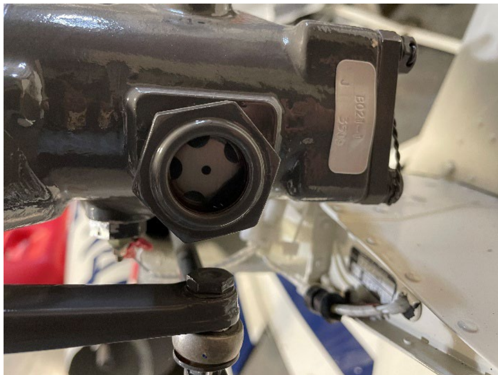
Figure 3. View of tail rotor gearbox oil level sight gage.
