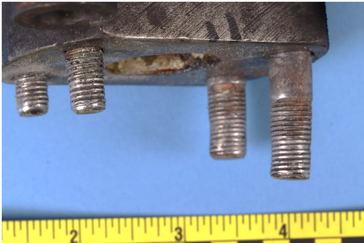
Figure 7. Closer aft view of the bolt threads in Figure 6, showing deformation.
