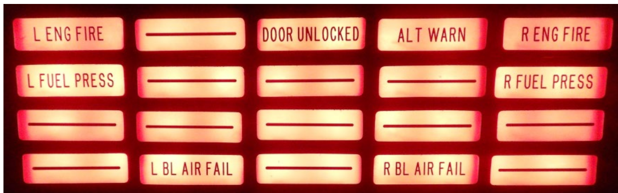
Figure 6: The annunciator panel test switches
