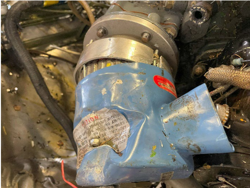
Figure 6. View of alternator prior to removal from engine.
