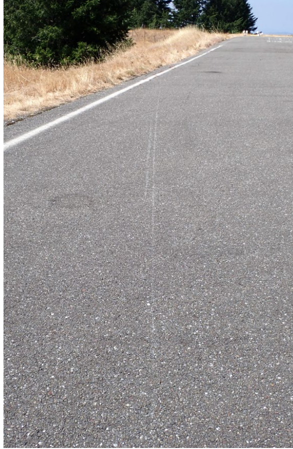
Figure 5: Long white runway contact mark
