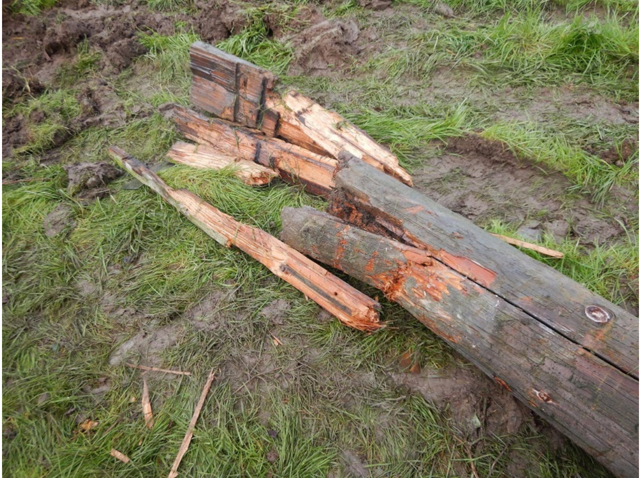
Figure 6. Top and middle section of the support pole showing white color transfer on the middle section.
