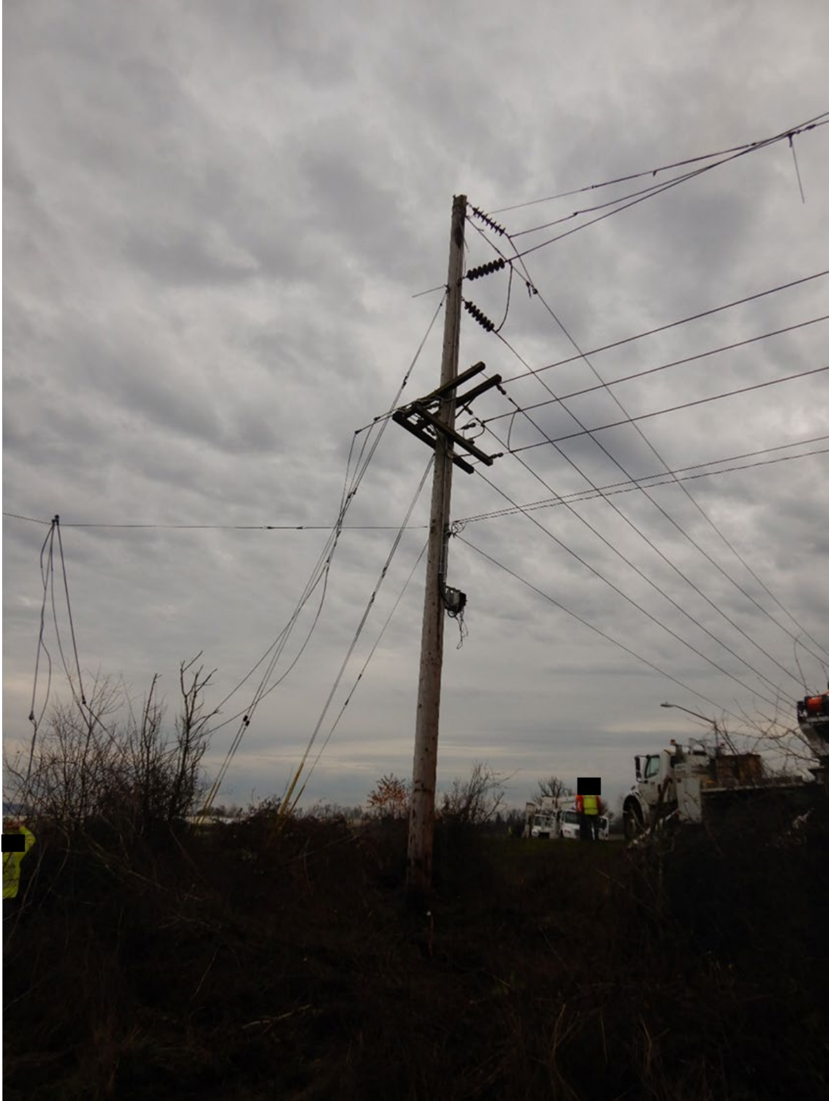
Figure 3. Support pole that was struck by the airplane.
