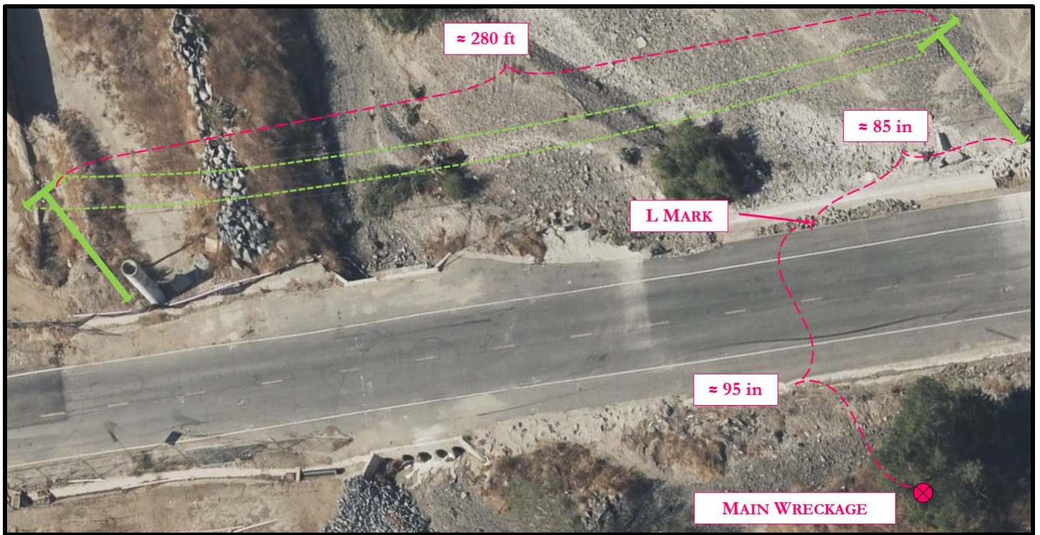
Figure 7: Accident Site in Reference to the Powerlines
