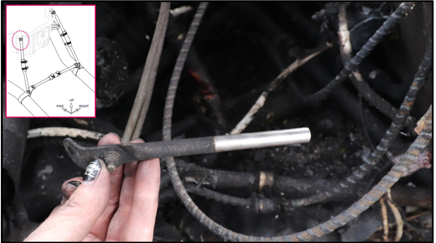
Figure 36: Exhaust Brace (loose)
