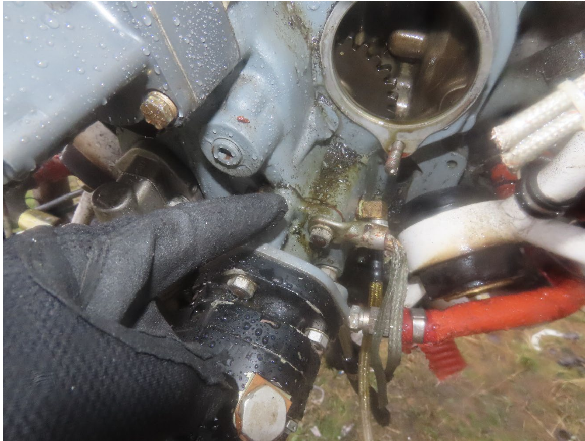
Photograph 5 - Engine oil pooling above and adjacent to propeller governor adapter and air/oil separator oil return line
