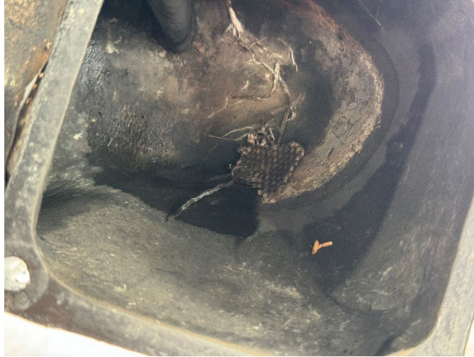
Figure 2: Remains of the high temperature cloth in the induction system.
