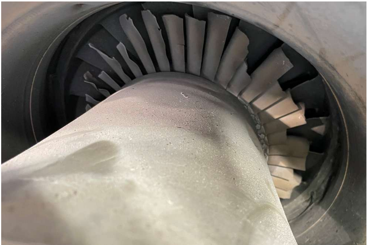
Figure 9. Damage observed on the No. 1 engine power turbine blades viewed through the exhaust.
