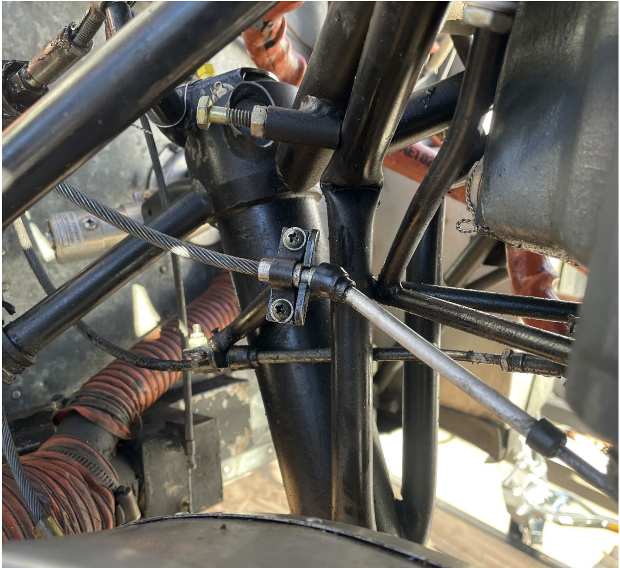
Figure 5-Throttle and mixture cable attachments and damaged engine support structure.
