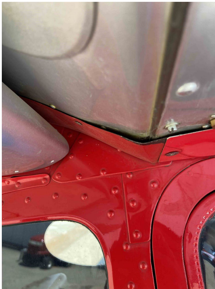
Photo 2 – View of structural damage (Courtesy of FAA)
