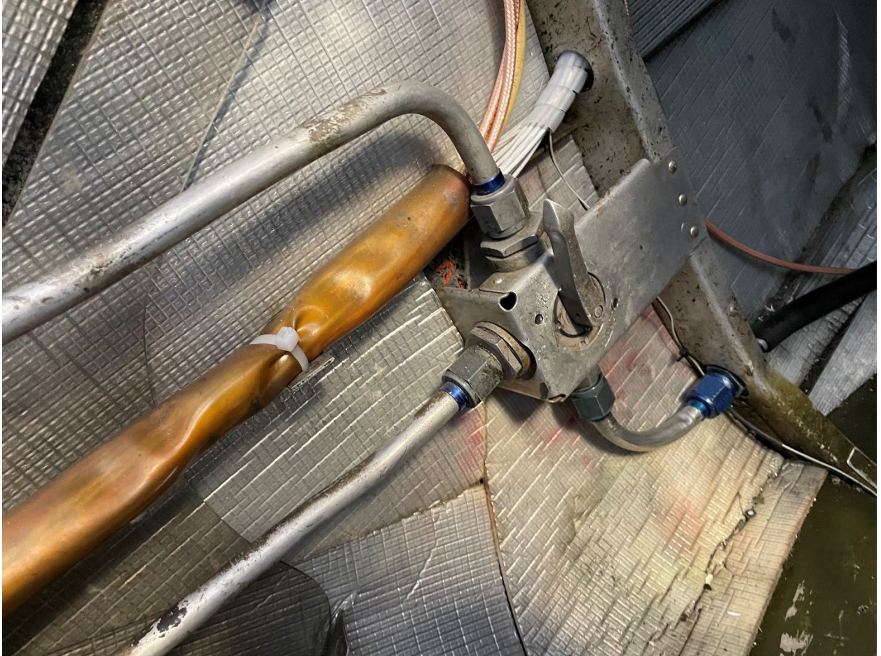
Figure 12. Fuel tank selector switch
