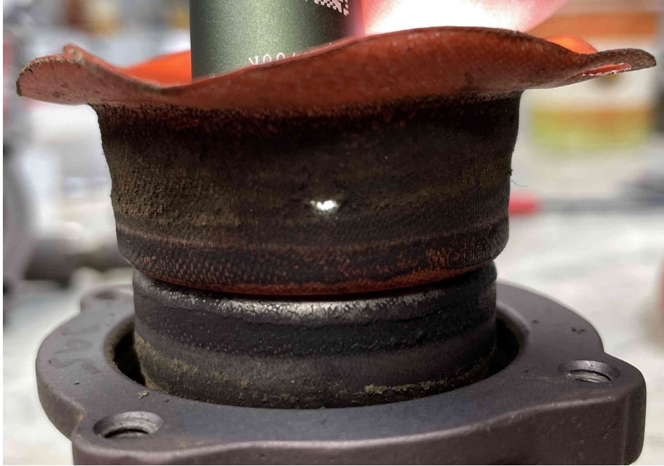
Figure 7 - Hole in diaphragm viewed from the outside - Engine #2.
