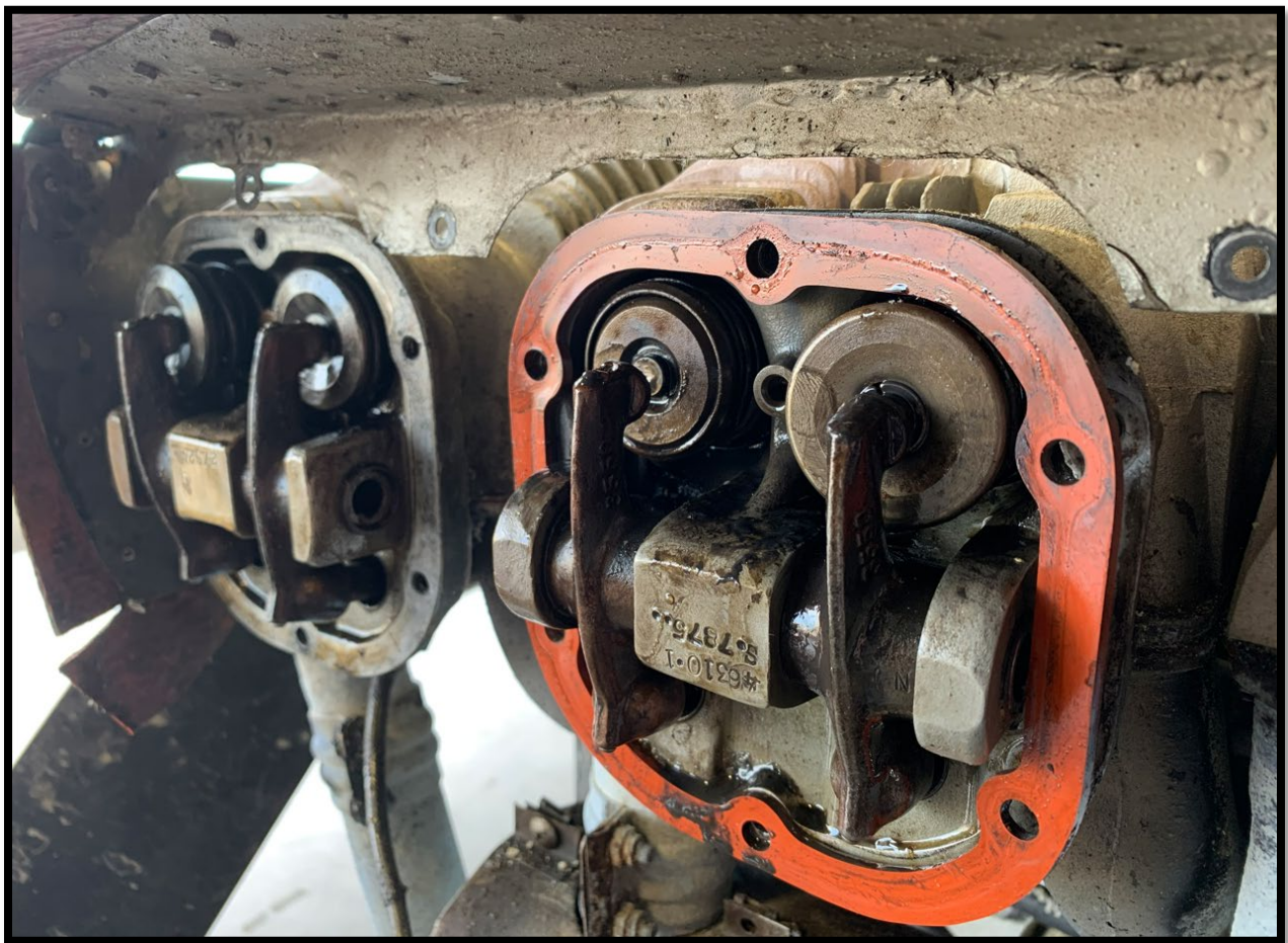
Figure 4. Cylinder no. 4 exhaust valve
