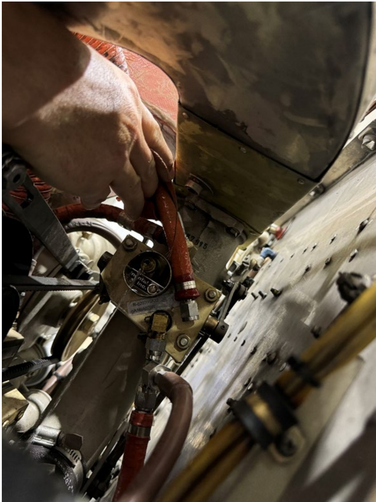
Figure 8. The fuel servo outlet line pulled away from the fuel servo.
