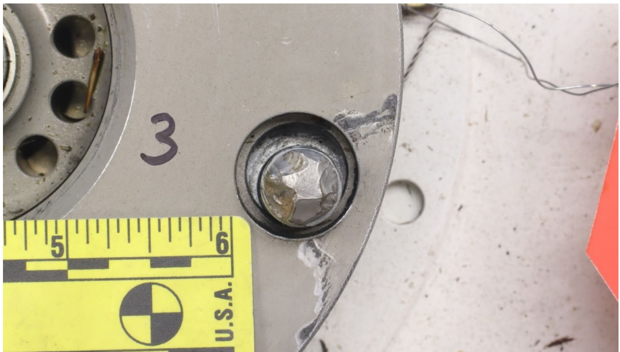
Figure 5. View of the fracture surface of the #3 bolt.
