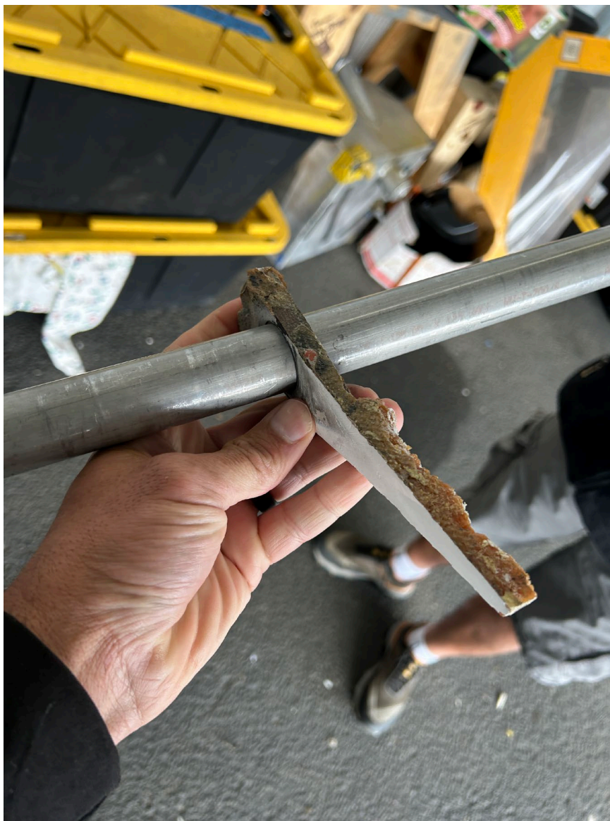
Photograph 4 - Outboard Trailing Edge Rib Upper Flange (Courtesy of Pilot)
