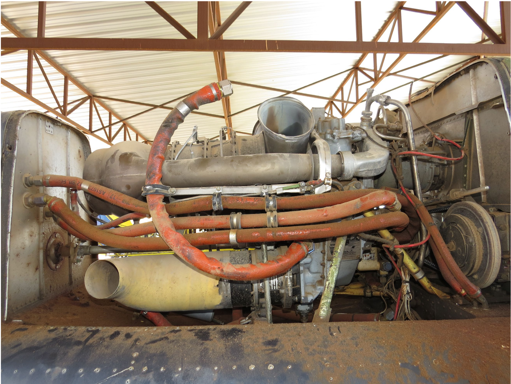
Photo 4 – View of engine prior to removal
