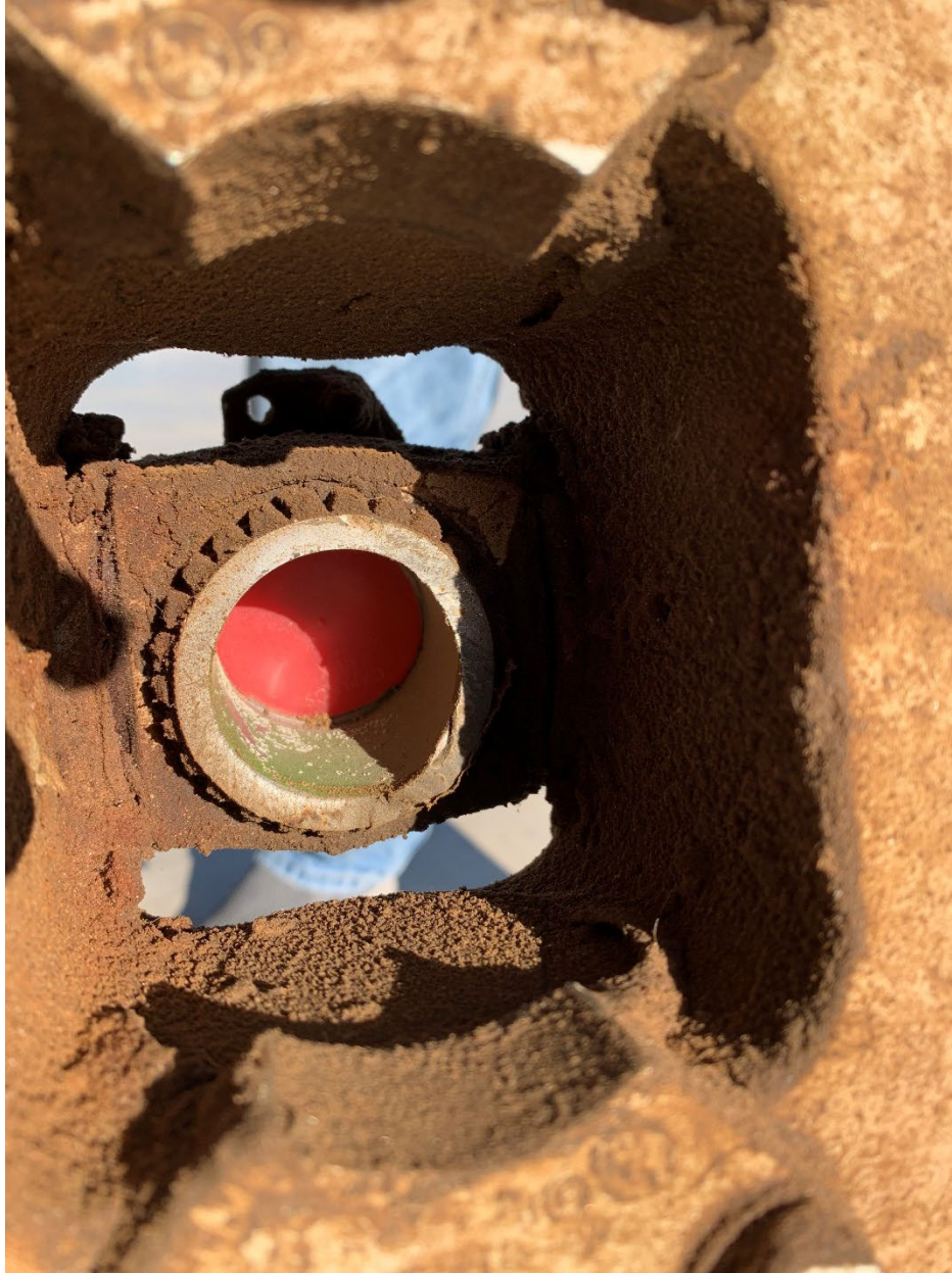
Figure 11. Upper section of mast in yoke.
