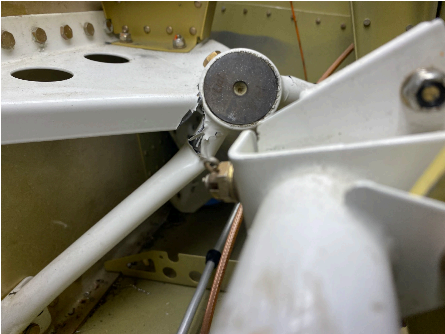
Photo 2 – View of Damage to Gear Mounts (Courtesy of the FAA)
