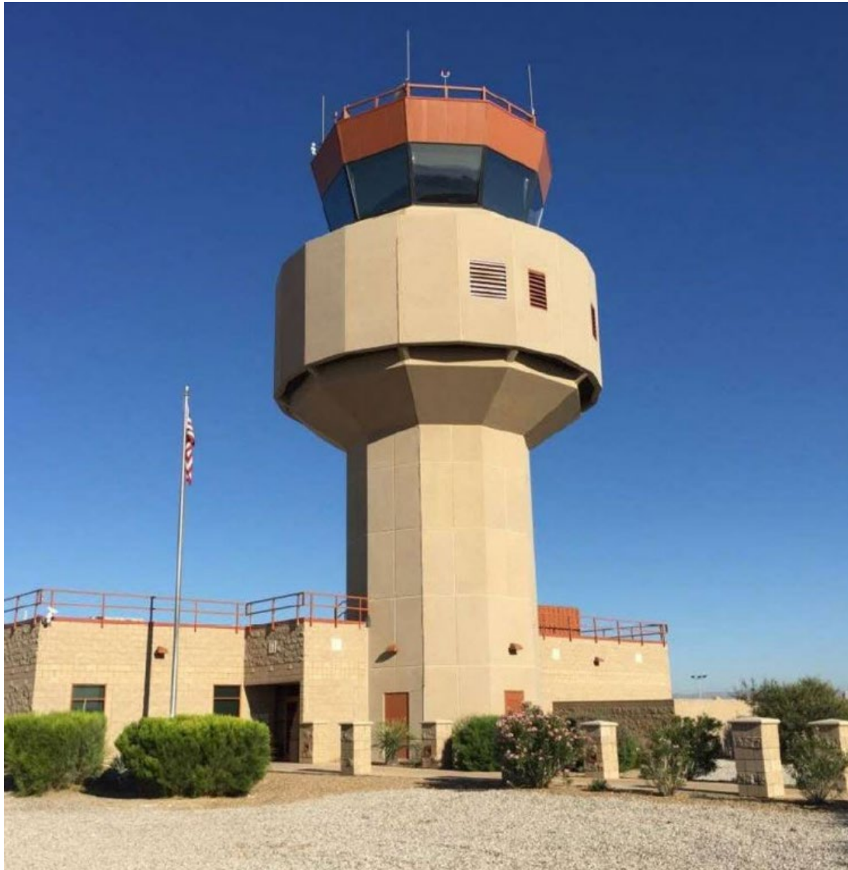
Figure 5. Photograph of the VGT airport traffic control tower.
