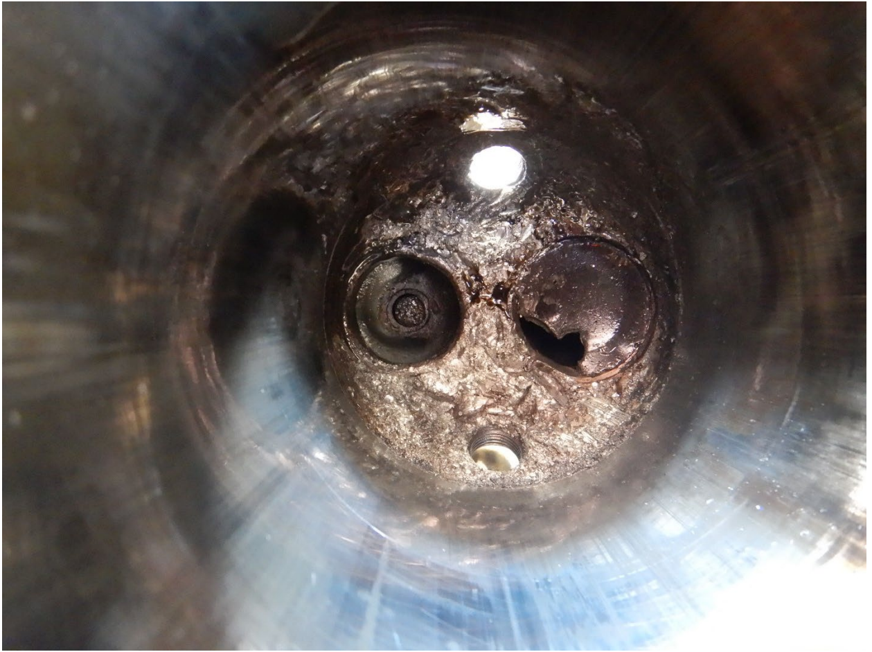
Figure 5 - No. 1 Cylinder Interior
