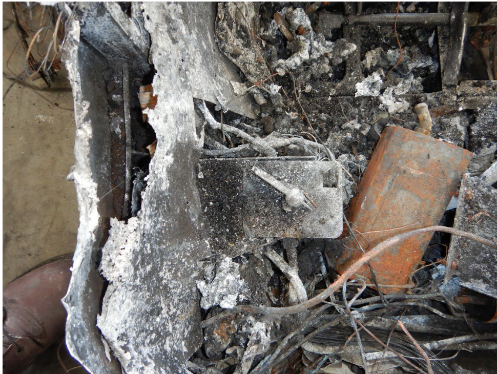
Photograph 5: Fire damaged fuel selector
