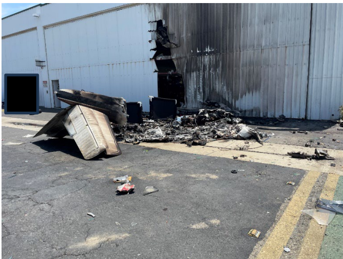
Photo 1 - View of Main Wreckage
