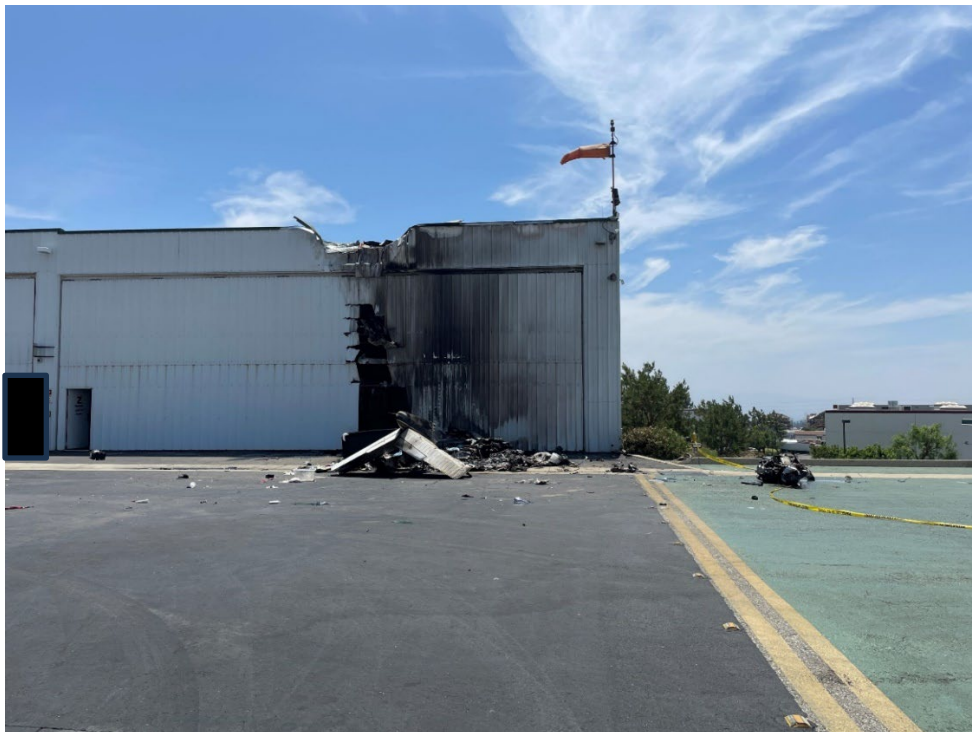
Photo 3 - View of Main Wreckage
