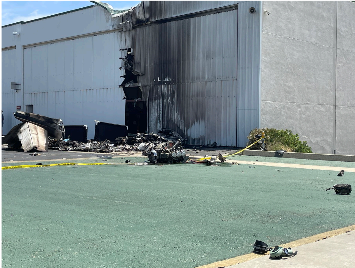
Photograph 2 - Overview of Main Wreckage
