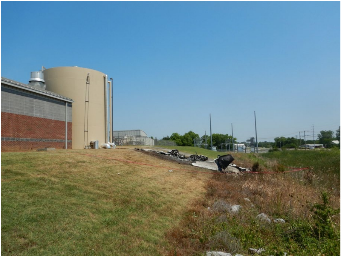
Figure 1: View of accident site north view
