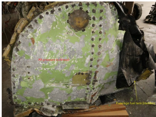
Figure 4. Aft pressure bulkhead.
