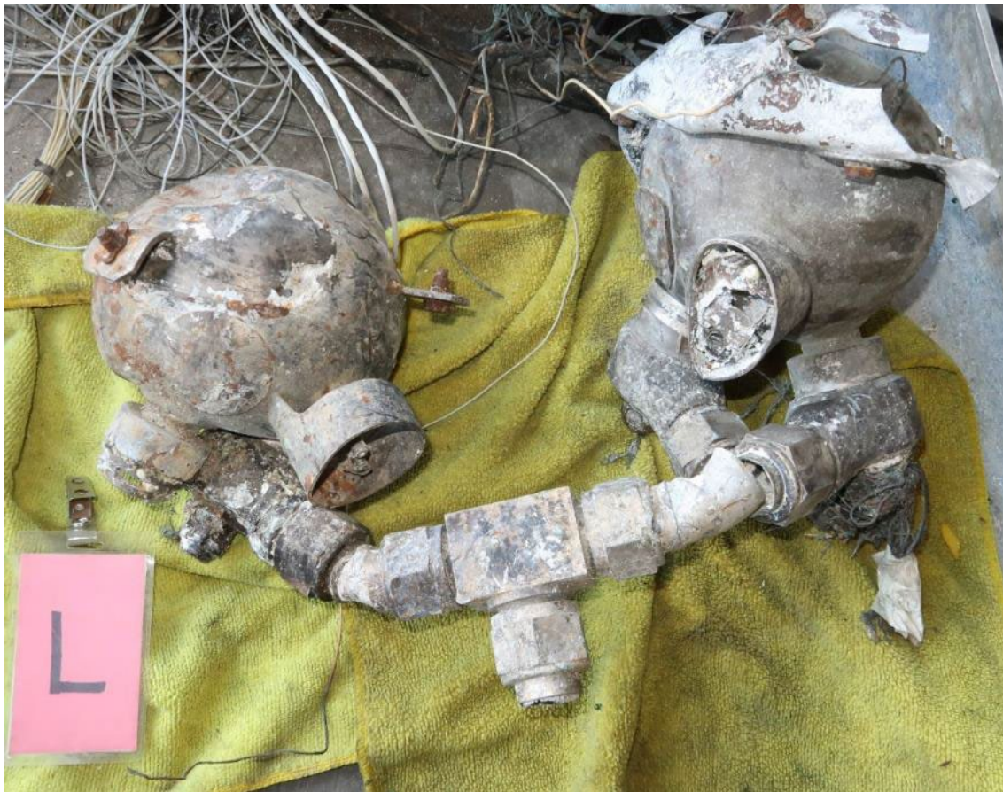
Figure 31. Fire extinguishing bottles.
