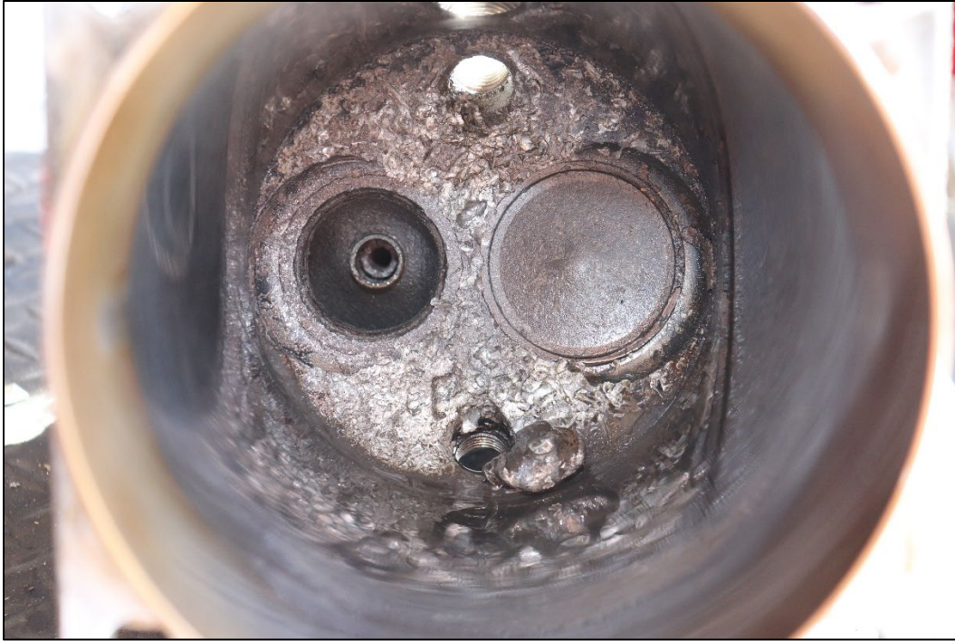
Figure 8: Interior view of number 4 cylinder
