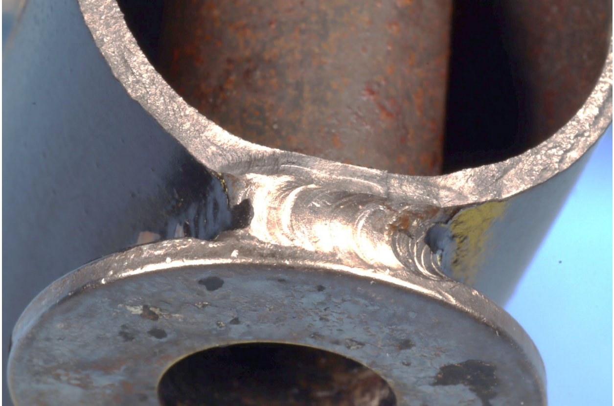
Figure 3. Fracture surface 1 exhibiting a thumbnail shaped fatigue crack and ratchet marks.
