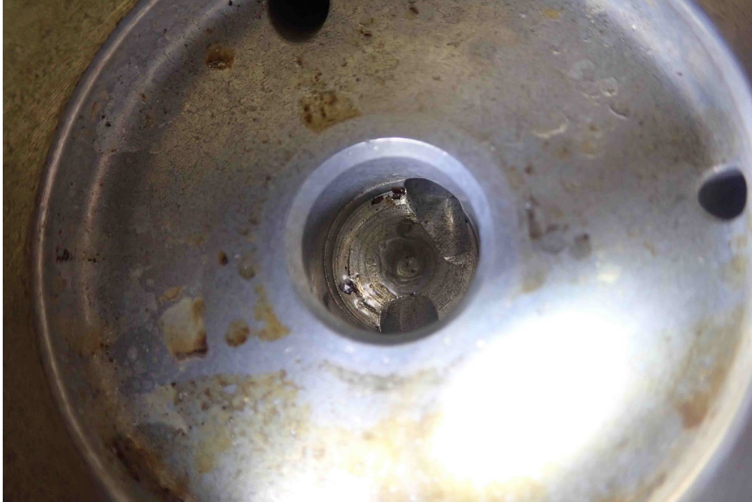
Figure 8 - Corrosion deposits on the servo valve seat cavity
