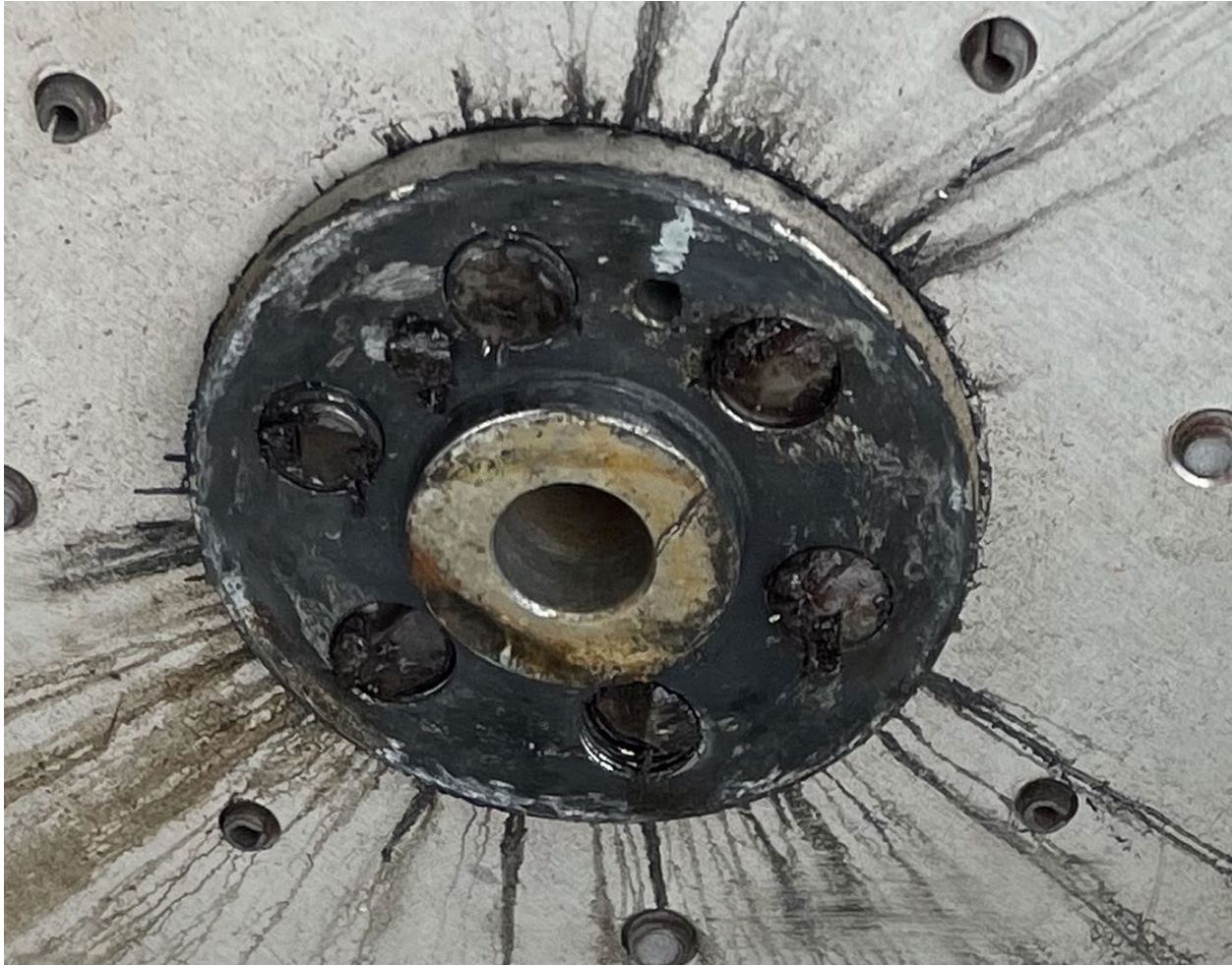
Figure 8. Close-up view of damaged cap bolts
