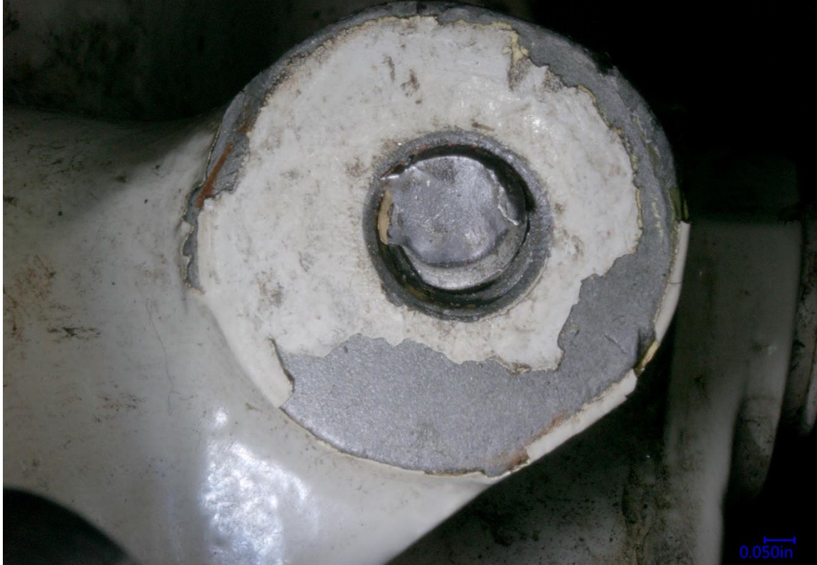
Figure 12. Closer view of the fractured bolt and surrounding housing.
