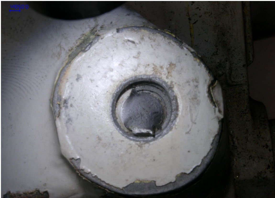
Figure 15. Closer view of the fractured bolt and surrounding housing.
