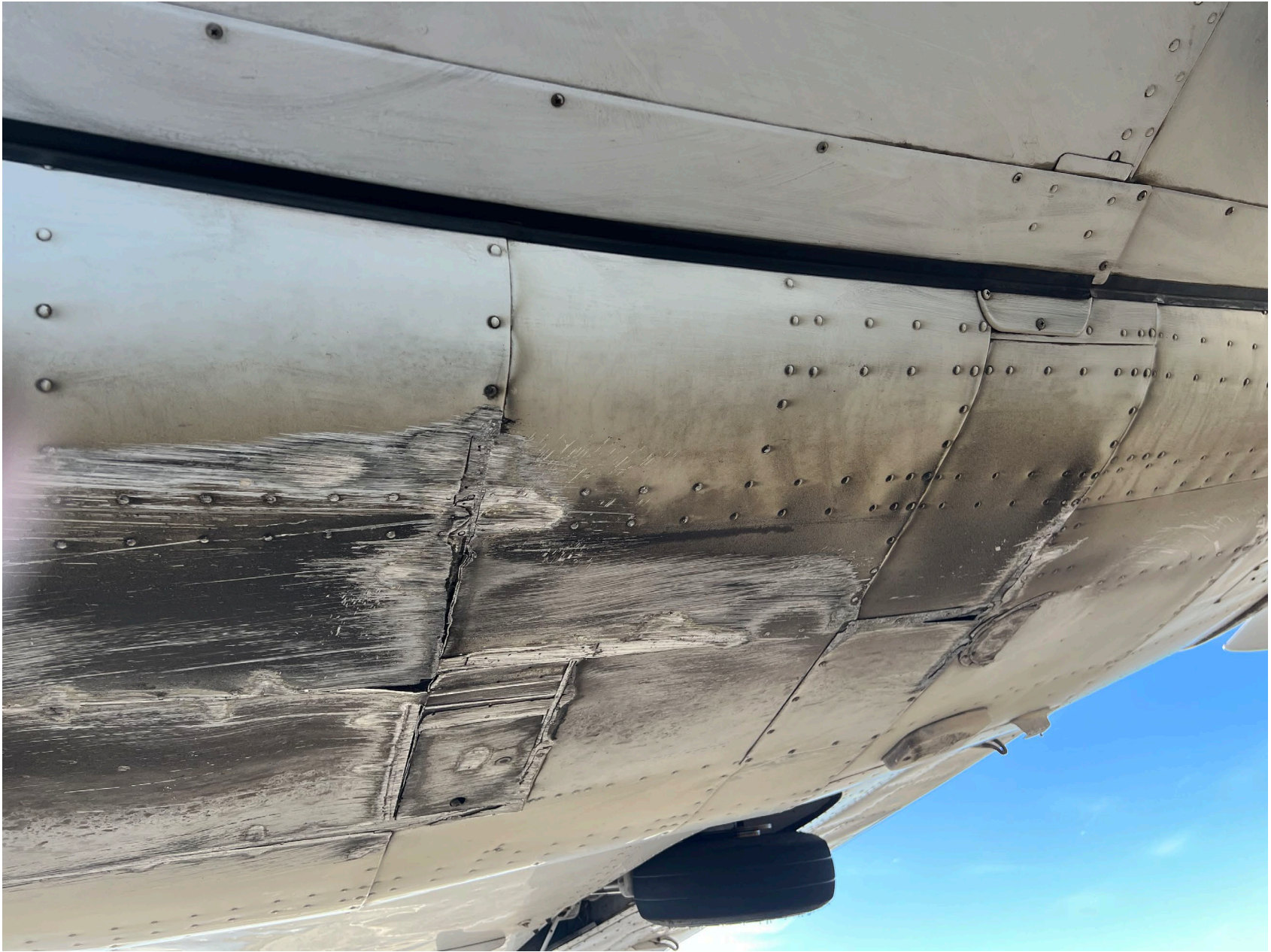
Photo 1 – Belly Damage (Strive Aviation Photo)
